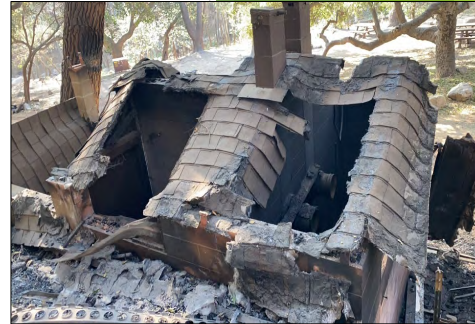
able Vault Toilet
